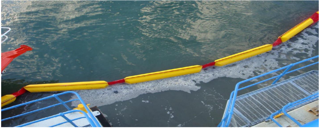
Figure 15 Example of a silt curtain surrounding marine construction works
